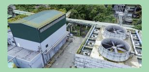
Following renovation completion and grid connection in February 2025, power generation per metric ton of clinker, under normal operation, increased from 14.89 to 32.33 kWh/ton. Control parameters are continuously optimized to minimize purchased electricity.
